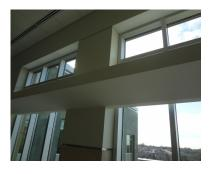
• Light shelves are used to make a room brighter making the most of sunlight entering the building. Horizontal shelves allow daylight to enter the building and reflect it throughout the space. This also decreases energy use because fewer light bulbs are needed.
