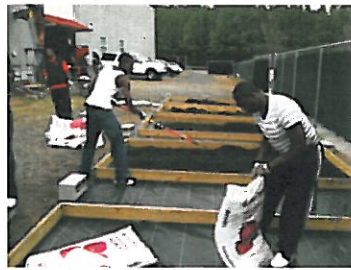
The students have installed the nursery fabric and are filling the raised beds with soil.
