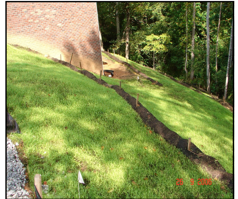
COMPLIANT GROUND COVER WITH MULCH WADDLES
