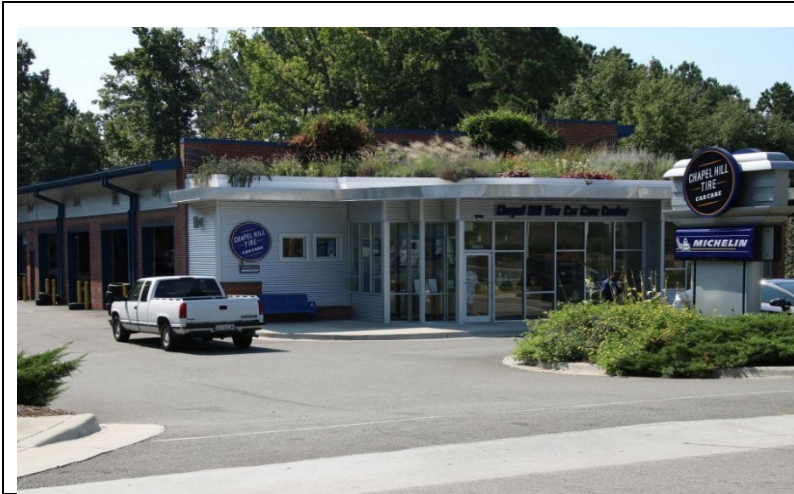
MA 71 SERVICE GARAGE
