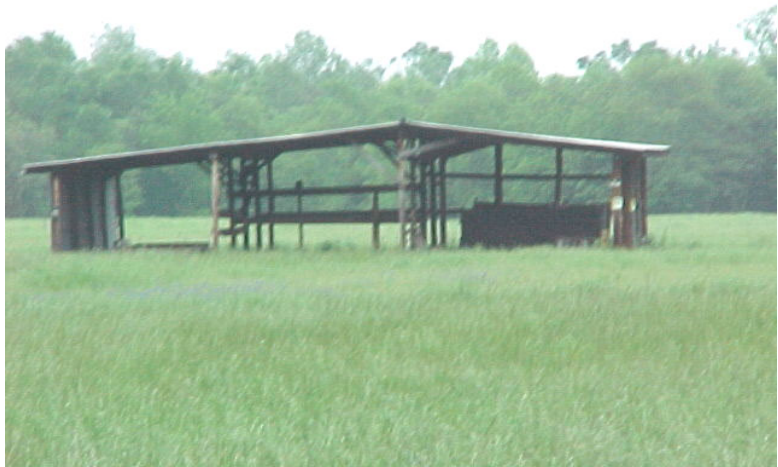
MS 15 POLE SHED
