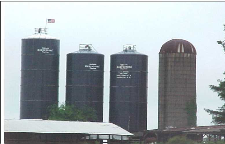
MS 28 SILO CON.STAVE AND GLASS LINED
