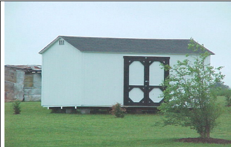
MS 17 STORAGE BUILDING
