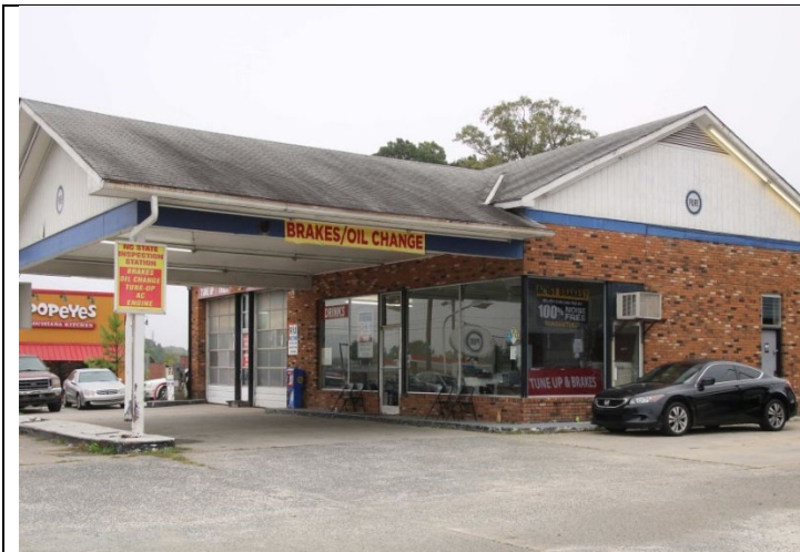
MA 73 SERVICE STATION
