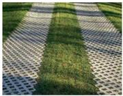
**PERMEABLE PAVEMENT** - Permeable pavement, an alternative to conventional concrete and asphalt paving, allows runoff to soak back into the ground instead of running off. Permeable pavement can be used for driveways, walkways and low flow parking lots. These materials reduce runoff, decrease flooding, filter pollutants and recharge groundwater. *This BMP is only eligible as a component of impervious surface conversion.*
