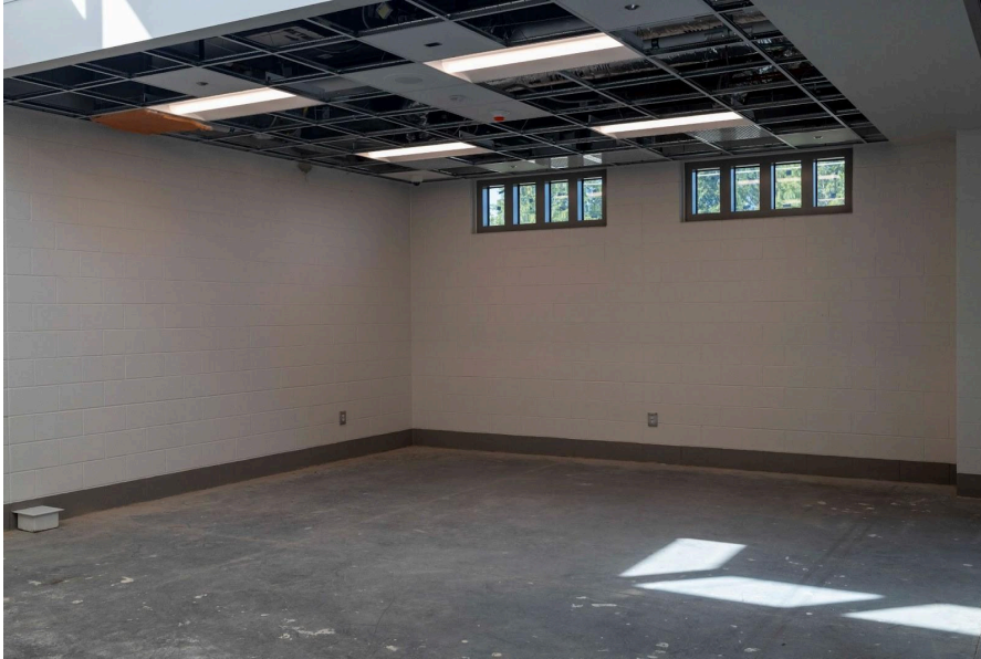
Location 4B - Classroom Interiors (1&2)
