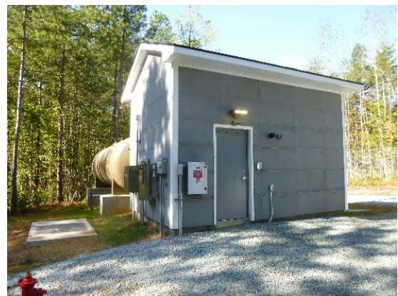
Rougemont Well House and Site Water System Number NC4032018
