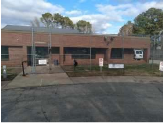
EXTERIOR VIEW AT ENTRANCE
