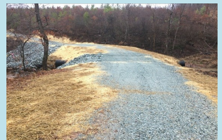
Road Repair picture
