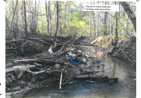
Existing conditions of stream
