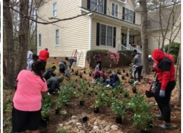
Students & teachers participating in the BETC program install a downspout disconnection and a critical area planting
