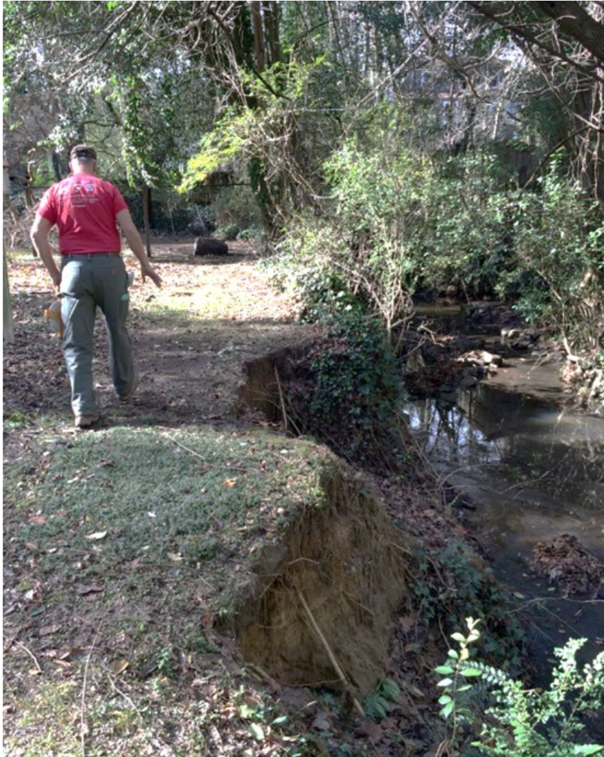
Below: Streambank stabilization - Before; several weeks after grading, matting, seeding, and planting with live stakes
