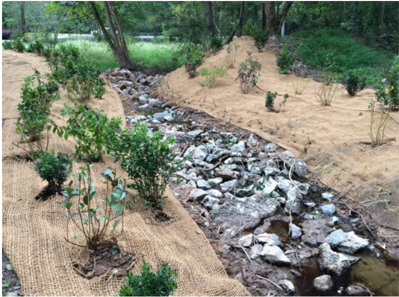
Below: Streambank stabilization projects - immediately after matting and planting; several months later
