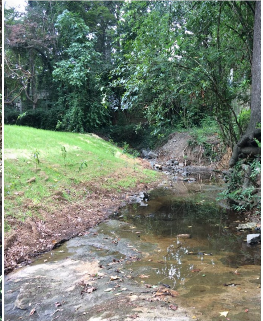
Below: Streambank stabilization - Before; several weeks after grading, matting, seeding, and planting with live stakes
