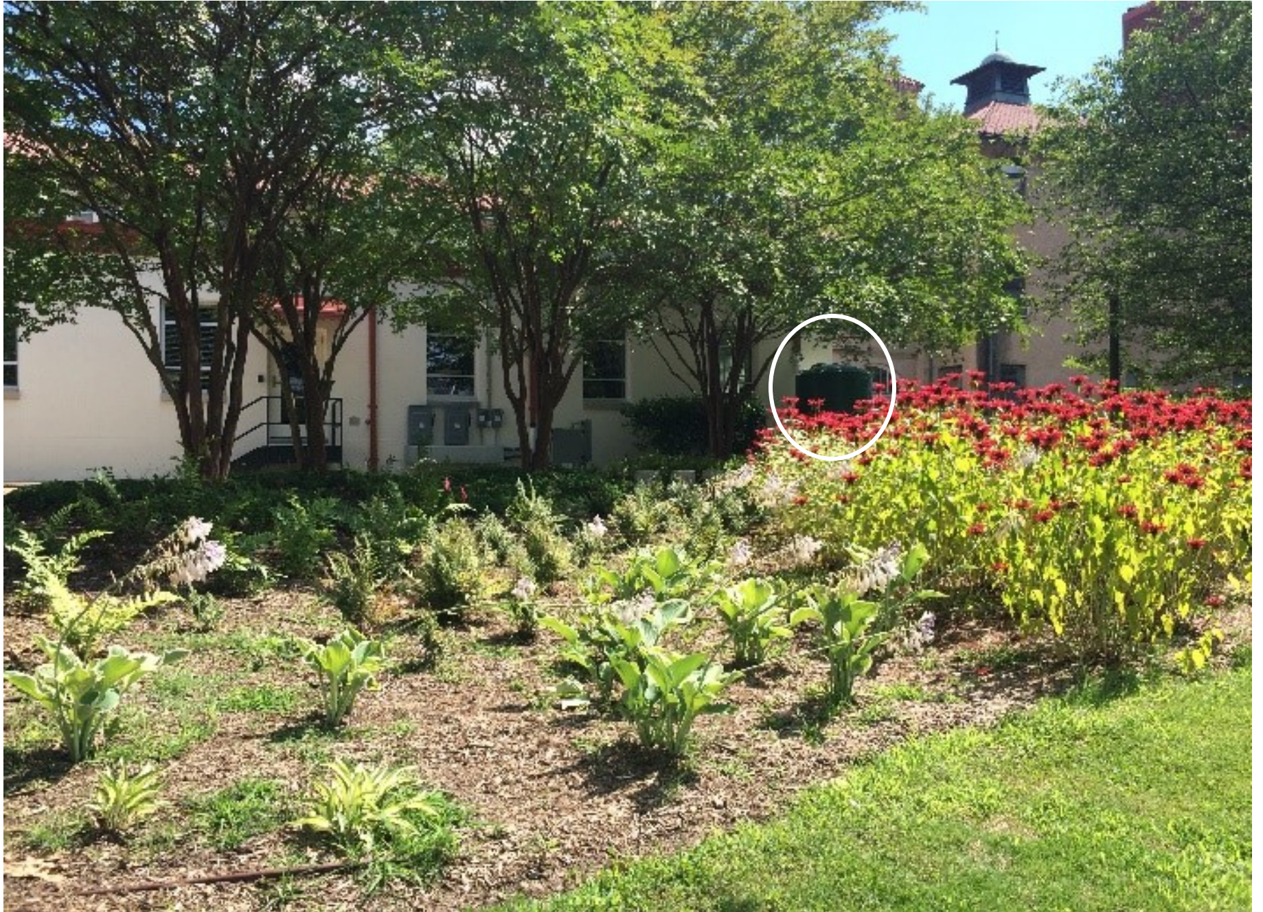
Below: Cistern (circled) at a school irrigating a critical area planting project (several months after cistern installation and planting).
