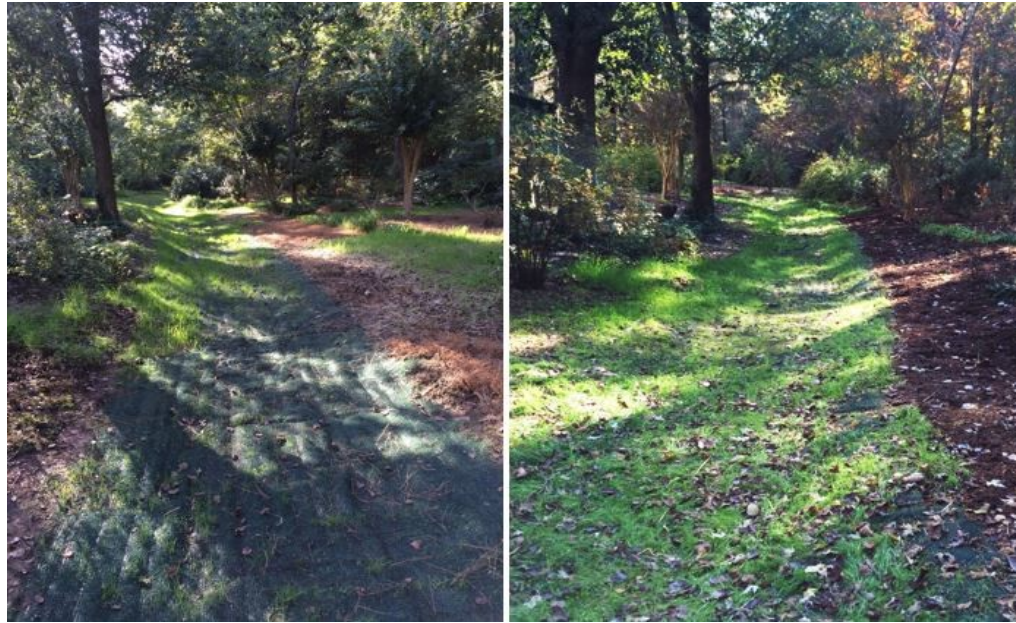
Below: Grass swale with Turf Reinforcement Matting (TRM); after 3 weeks
