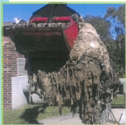
Example of a "Rag Ball" caused by "flushable" wipes and hair.
