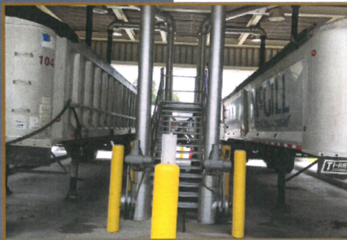
TWWTP's Sludge Loading Facility
