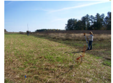
Pictured above: grassed waterway in progress
