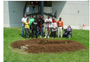
The students at Southern HS help install a rain garden at their school.
