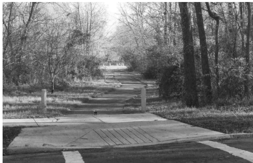
Bollards (with central bollard down for maintenance access) and accessible ramp onto North/South Greenway at W. Markham Avenue
