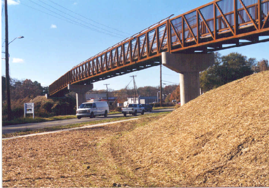
Lakewood Avenue bridge on the American Tobacco Trail
