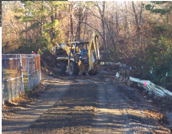
Work on the Rocky Creek Trail in 1999
