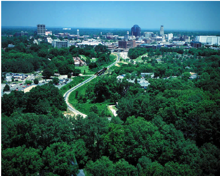
The ATT from the south, looking towards downtown
